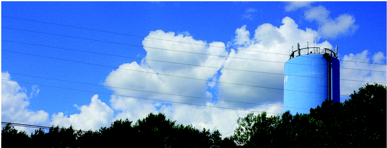
Bancroft water tower
